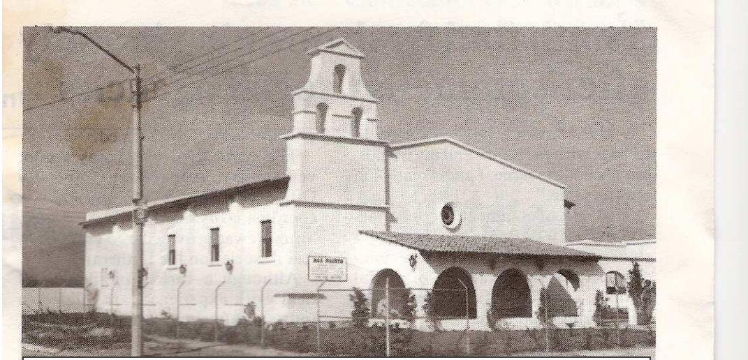
GUADALAJARA-The new building for All Saints Lutheran Church in Guadalajara, Mexico represents a turnabout from a near dead congregation to one that anticipates a bright future.
