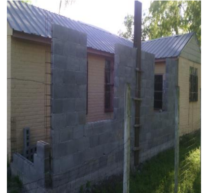
New wall at Bethel in Rio Rico
