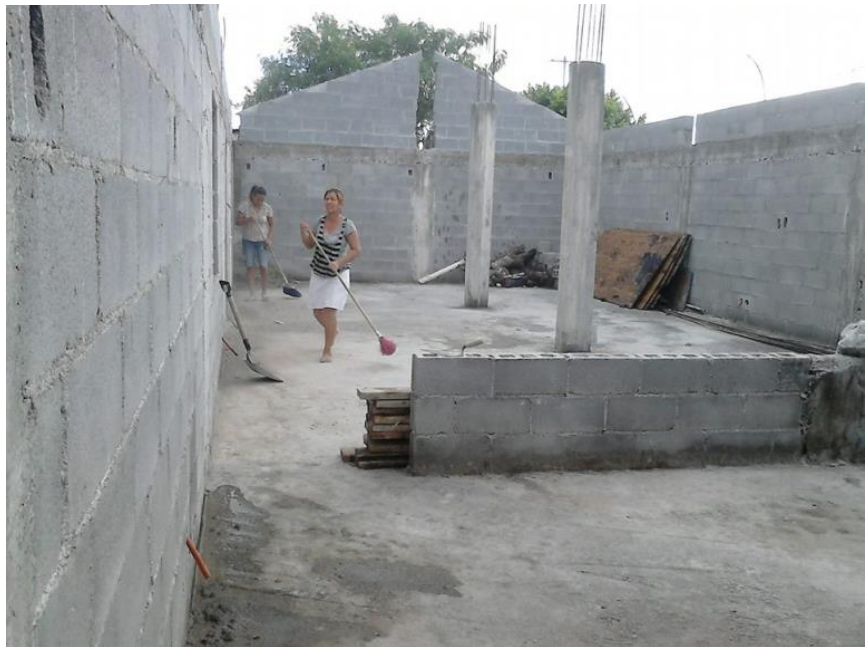
A view of the church from front to back. The short wall in front will be where the chancel area will be.
